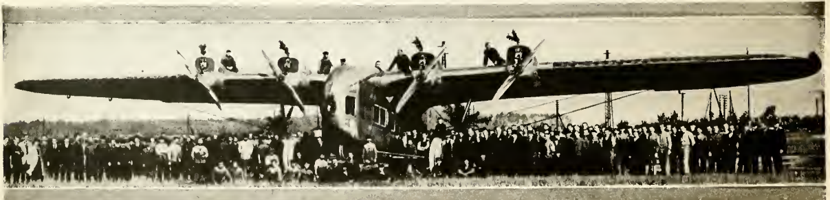
The Rohrbach "Staaken," a 1,000 h.p. multi-engined all-metal 20-passenger monoplane built in 1920
